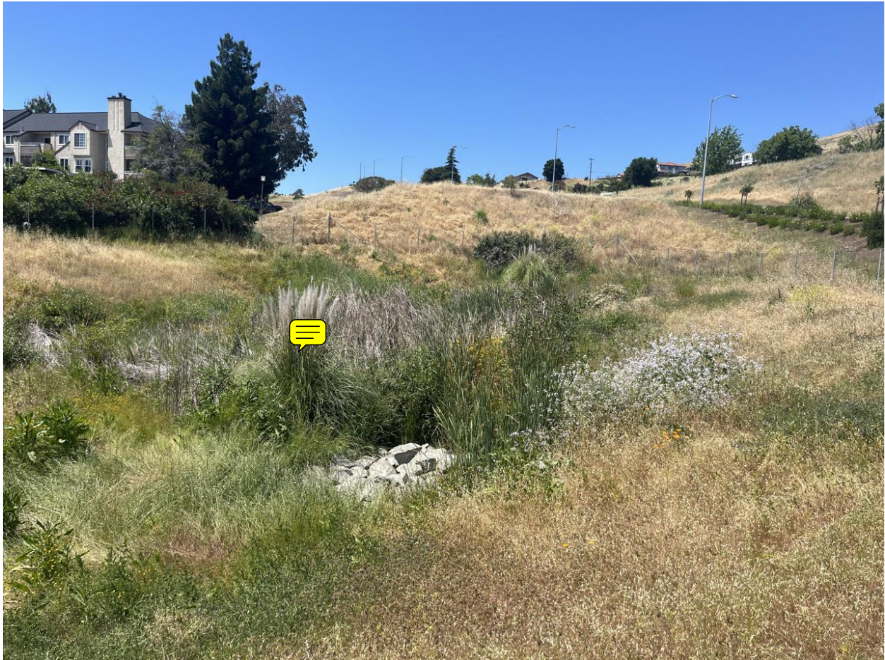
PHOTO 2: Site Condition B – Alquire Water Retention/Detention Facility with Overgrown Vegetation
