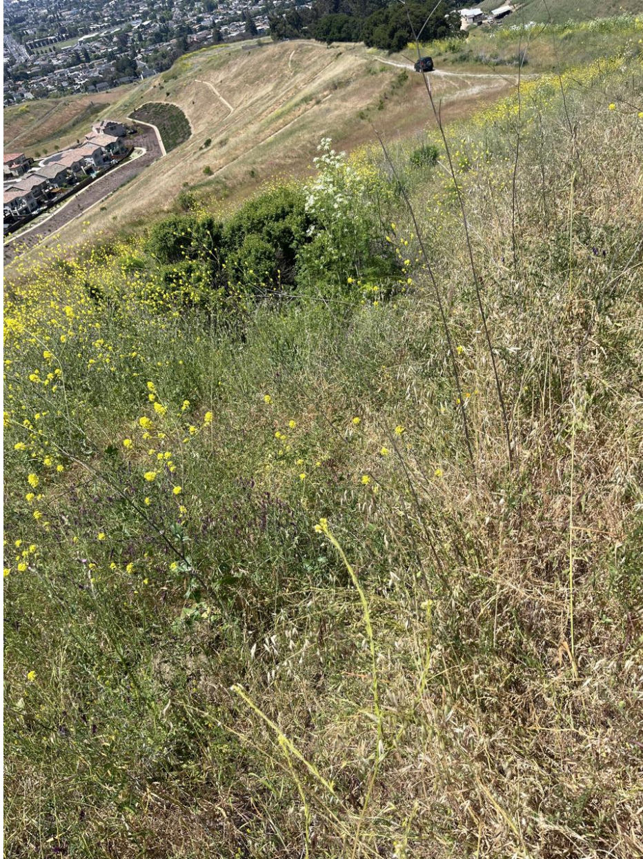
PHOTO 1: Site Condition A – Scarp Development adjacent to the Access Road
